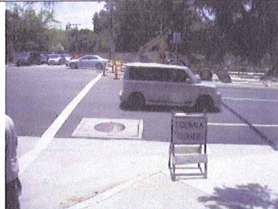
This was taken the day after the risk assessment. As noted ""SIDEWALK CLOSED" signs had been set up on both the north and south entrances.
